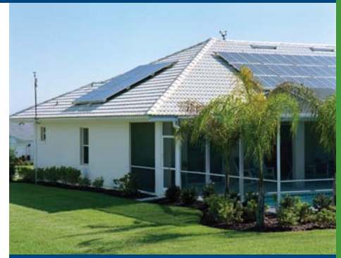
Solar Thermal and PV Panels, Lakeland House, Lakeland, Florida
