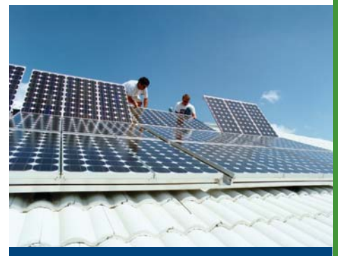
Installation of PV Panels, Lakeland House
