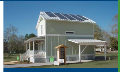
PV panels on the Callaway House
