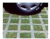
A sub-base consisting only of sand and gravel will have less ability to support grass roots growing into it. This restricts the grass root zone primarily to the topsoil directly above the sub-base, and can be subject to more rapid drying out in drought conditions. Including soil in the mixture of sand and/or gravel will permit better growing conditions for the grass.
